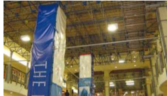
The overhead protective structure used in the Broadway expansion.
